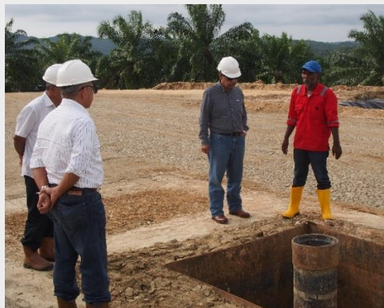
AMT-1 location with Operator GM, Drilling Mgr and site contractor
