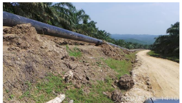
New gas pipeline under construction through SBA – Passing close to the Paya-Bili Lead
