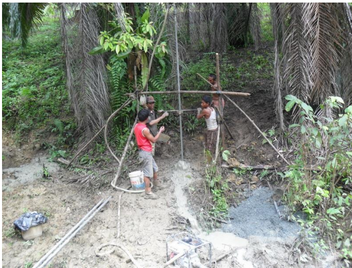
Shallow oil wells being hand drilled by locals on flank of Simpang Lead
